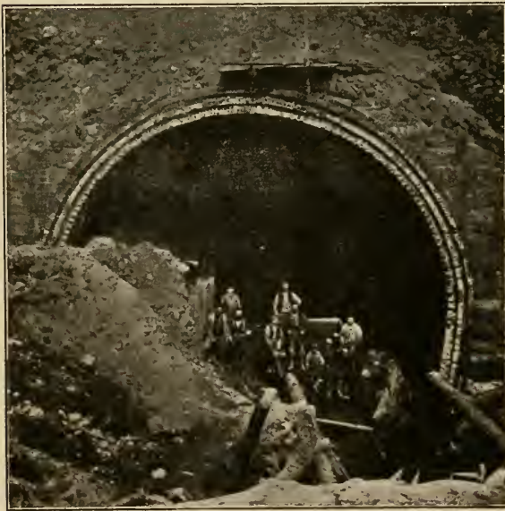
HOOSAC TUNNEL UNDER CONSTRUCTION, 1871
